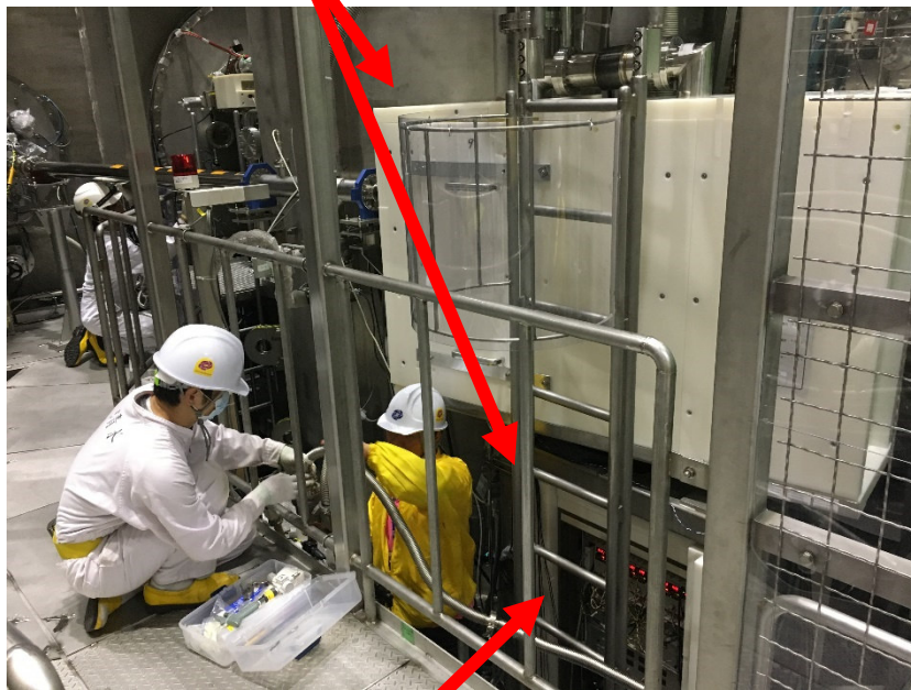
Power supply, vacuum gauge controller, etc.
