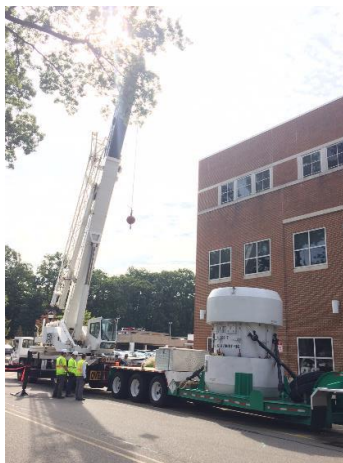
FIG. 4. The Crane and the Cask in the parking lot behind the hospital
