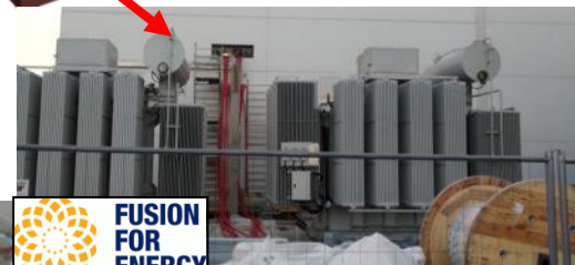
AGPS Conversion system 60MW CW
