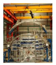
Figure 5 : OIS installation onto a TF coil
