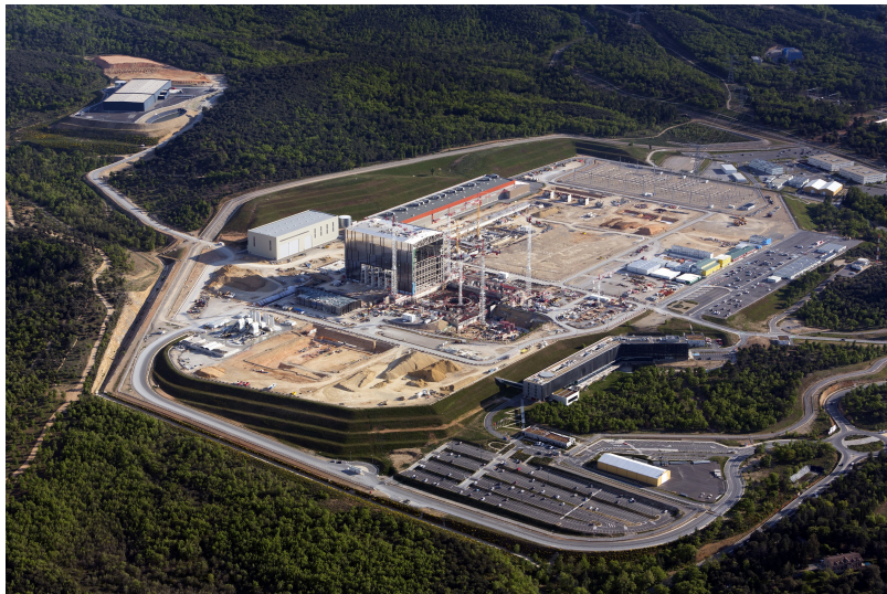
FIG. 1: Aerial view of the ITER site at St-Paul-lez-Durance with the construction of the Assembly Hall and Tokamak Complex in the centre of the photograph. The circular form of the bioshield, which will house the cryostat and tokamak core, can be seen in the centre of the Tokamak Complex. A large logistics warehouse can be seen on the hill above the main site.
