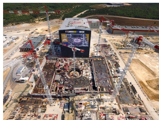
FIG. 3: A view of the Tokamak Complex construction with the Assembly Building behind. The Tokamak Building is in the centre, with the form of the circular Tokamak Pit (inner diameter ~30 m) visible; the Tritium Building is on the left and the Diagnostics Building on the right of the Complex.
