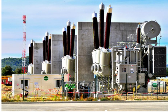
FIG. 12: Main 400 kV step-down transformers installed at the ITER site.
