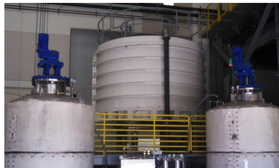
Figure 6. Completed VPI mold and resin pumping systems
