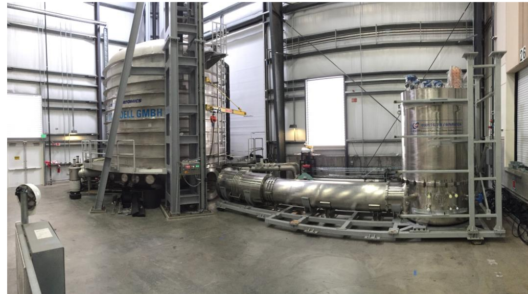
ASIPP provided HTS Feeder and Cryostat
