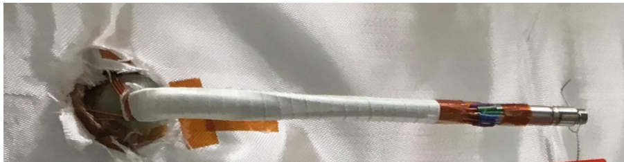
Quench detection wires and pipe after insulation
