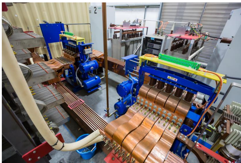
Redundant 50kA DC Breakers
