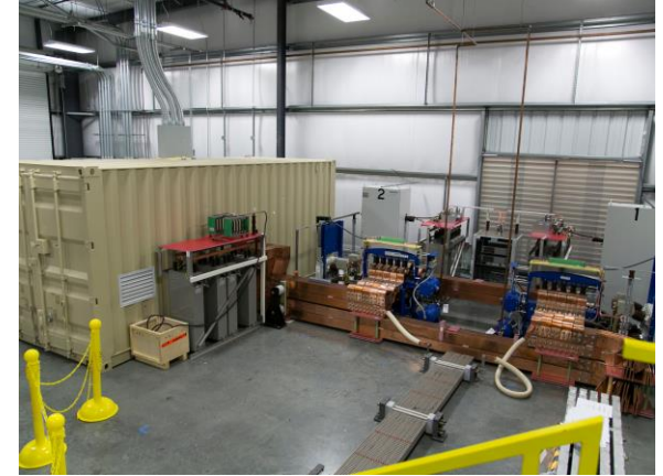
0.5 MW DC Power System
