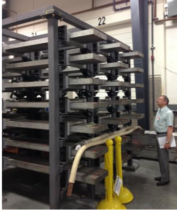
0.130 \Omega Dump Resistor
