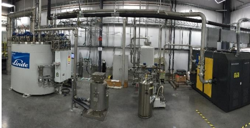
900W Liquid Helium Cryo System
