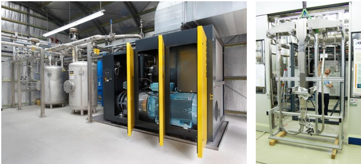
FIG. 2. Left:HELOKA-LP helium loop at KIT. Right: Double compartment prototype of the HFTM during installation
