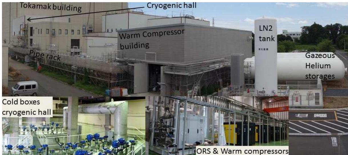
Fig.13: Composite view of the cryogenic system installed at Naka (ORS: Oil Removal System)
