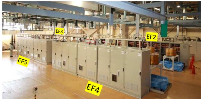
Fig.11: The EF power supplies during installation at Naka. (EF4 & EF5 in front of the picture EF2 & EF3 on the back)
