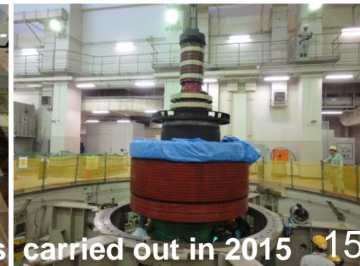
Overhaul of H-MG was
