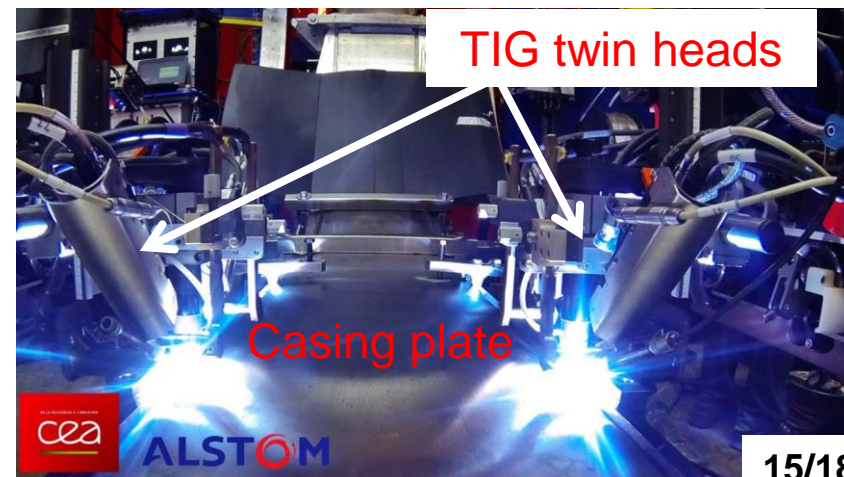
Longitudinal welding by TIG twin heads
