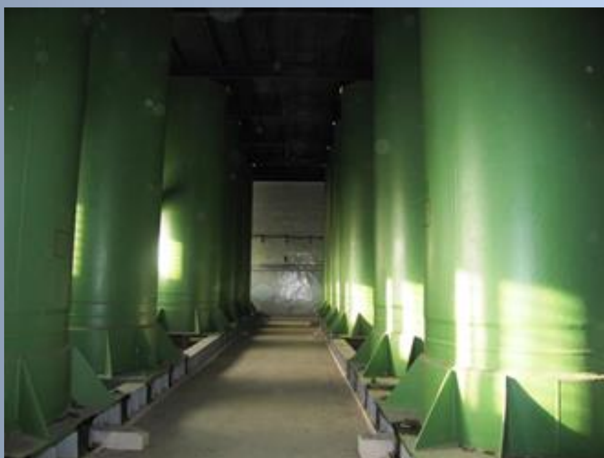
ECCS pressured tanks view in Building 117/1
