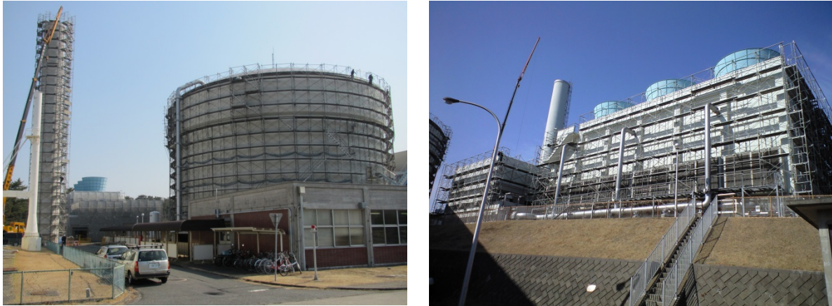
FIG.1. Repair of reactor building and cooling tower.
