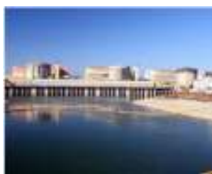
Cernavoda Nuclear Power Plant – ROMANIA
