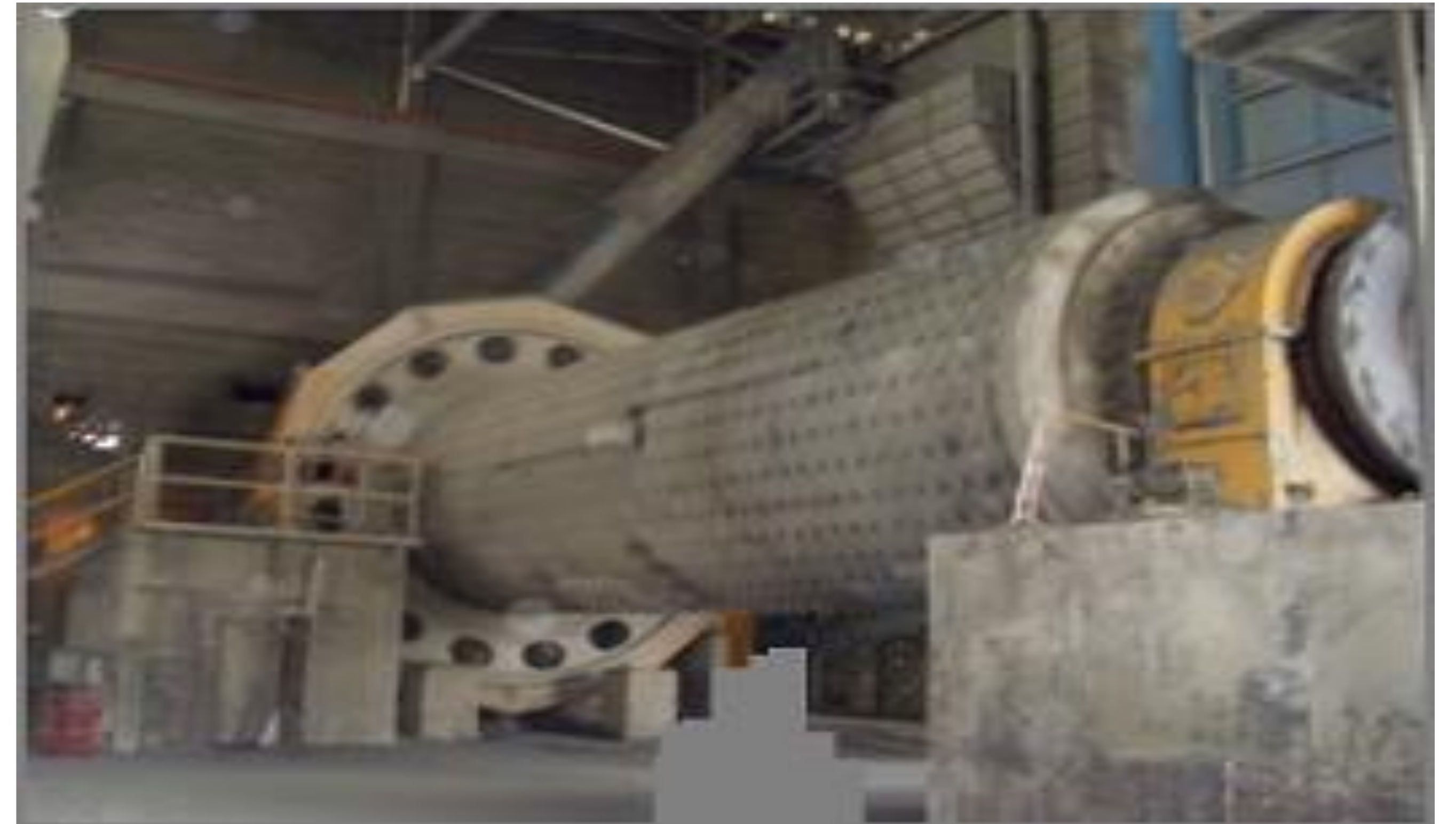
Figure 2. External View of the GHACEM Mill
