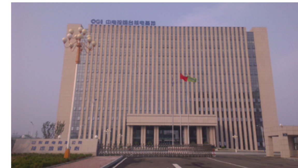
FIG. 5 Nuclear Emergency Material Store Basement of CPI in Yan Tai
