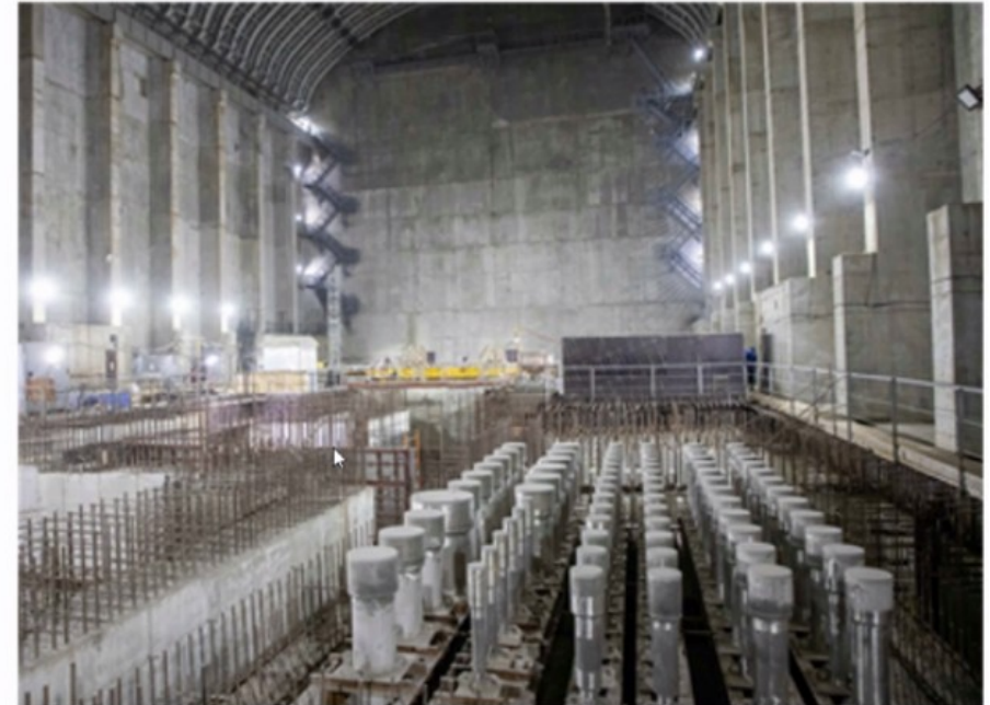
MBIR construction site (2024)
