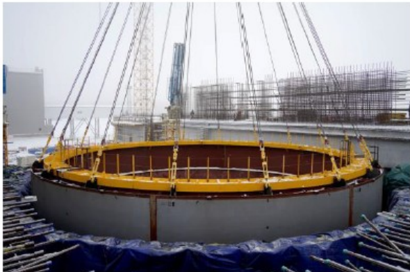
The lower tier of the enclosing structure was immersed in the reactor shaft (December 2023)
