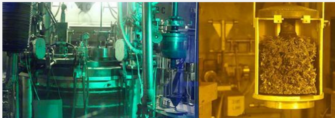
Illustration from: https://mfc.inl.gov/SitePages/Instruments/Fuel%20Conditioning%20Facility/Mark%20IV%20electrorefiner.aspx
