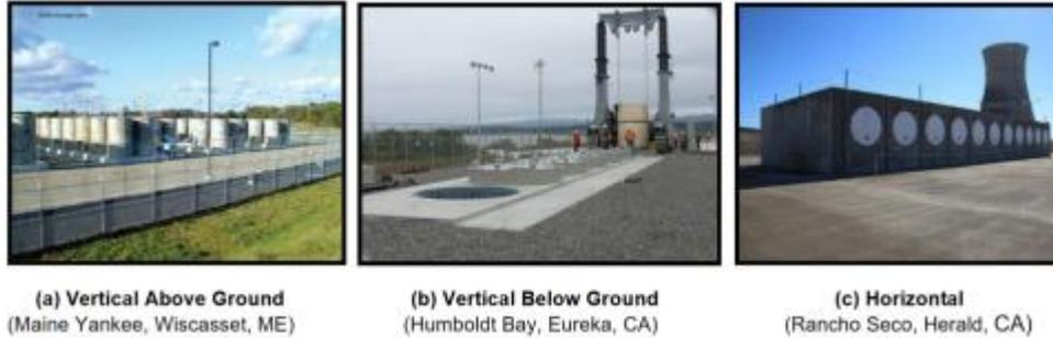
Figure 4-3 Dry Cask Storage Systems (Freeze et al., 2021; Recharad et al., 2015).
