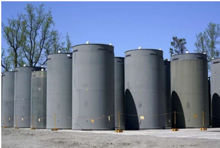
INTERIM DRY STORAGE FACILITY
