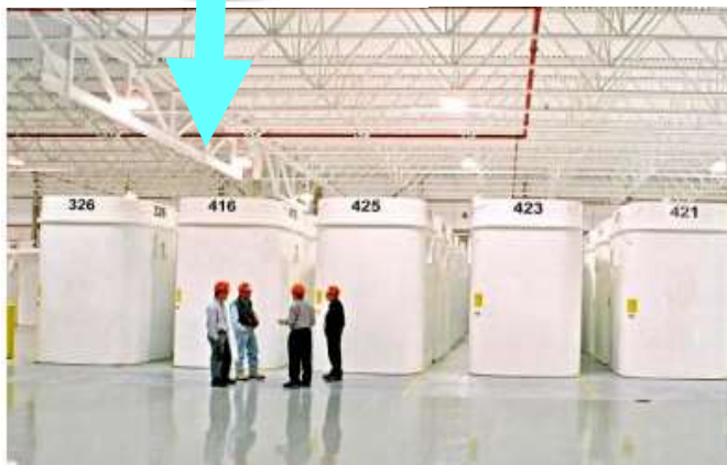
CASKS INTERIM DRY STORAGE
