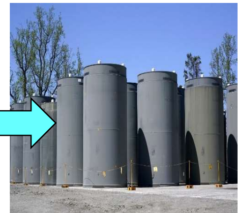
INTERIM DRY STORAGE
