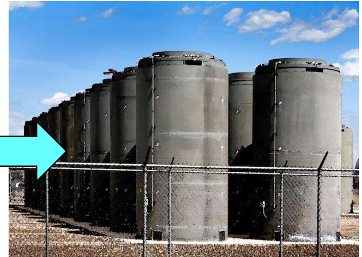
INTERIM DRY STORAGE
