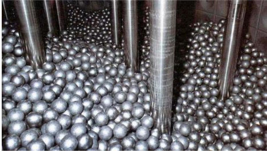
Figure - THTR reactor core with control rod bars
