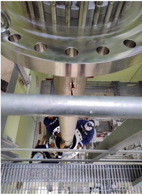
Axial flow pump installation
