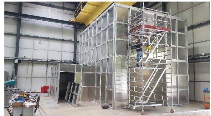
High voltage laboratory
