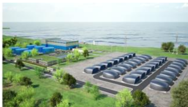
Artist's impression of an array of 32 modules configured in line with turbine hall, GridReserve® storage facility and sub-station
