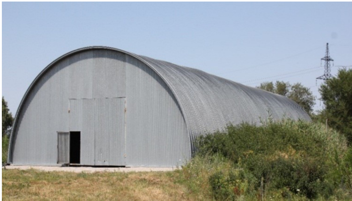
Low activity radioactive waste storage
