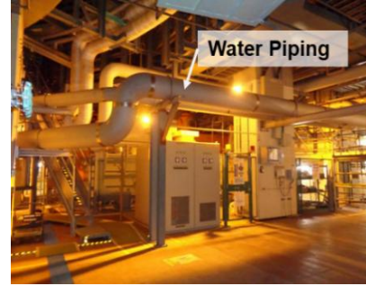
FIG. 8 Water piping installed under Tokamak-hall
