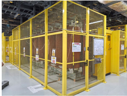
Figure 2: The European EC main HV power supplies installed in the level 1 of the ITER RF building occupying an area of around 16 x 20 m.
