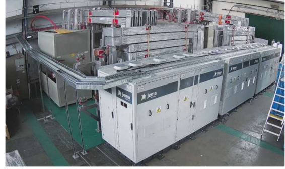
FIG. 3 Image of the TF power supply after assembly
