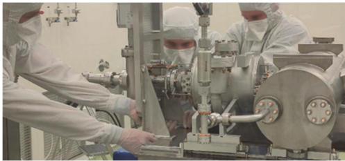
FIG. 9. Installation of the component of the beam line in the clean room.
