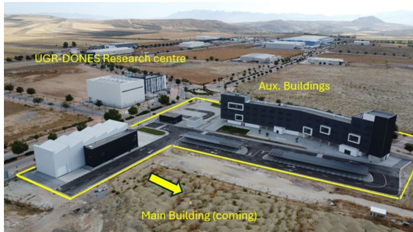
Figure 1. Current status of civil works on the IFMIF-DONES site
