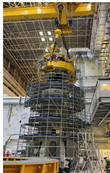
FIG. 2. The fourth CS module being stacked on CS Assembly. All 6 modules are now delivered from the US
