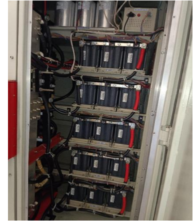
Fig-2: Super Capacitor bank Assembly
