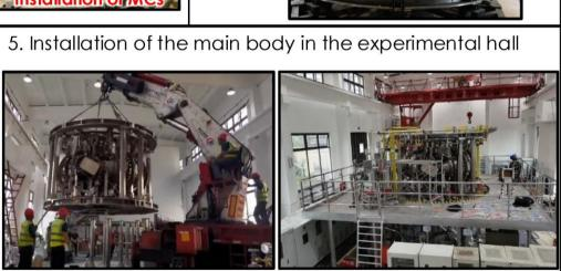
Maximum position deviation of the MC system including dimensional deviation is achieved to be less than ±3 mm measured by a laser tracker. It will not significantly affect the magnetic field configuration\*. \*G. Xiong et al., Plasma Phys. Control. Fusion 65 (2023) 035020.
