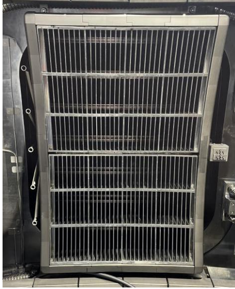
FIG. 4. Photo of the FAM launcher in HL-3. A gas puffing system with tree poloidal injections are located at the left of the launcher mouth (as viewed from the plasma). A set of Langmuir probes is located to the right.
