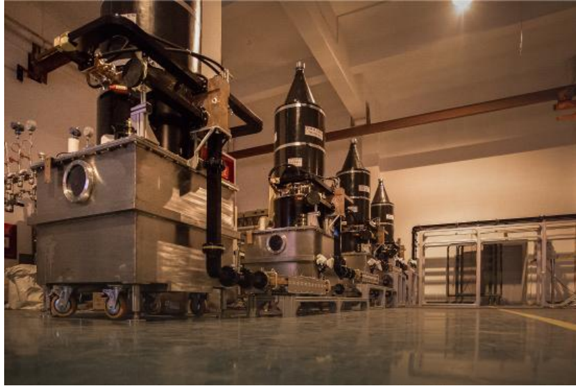
FIG. 2. The Klystrons installed in the RF heating hall
