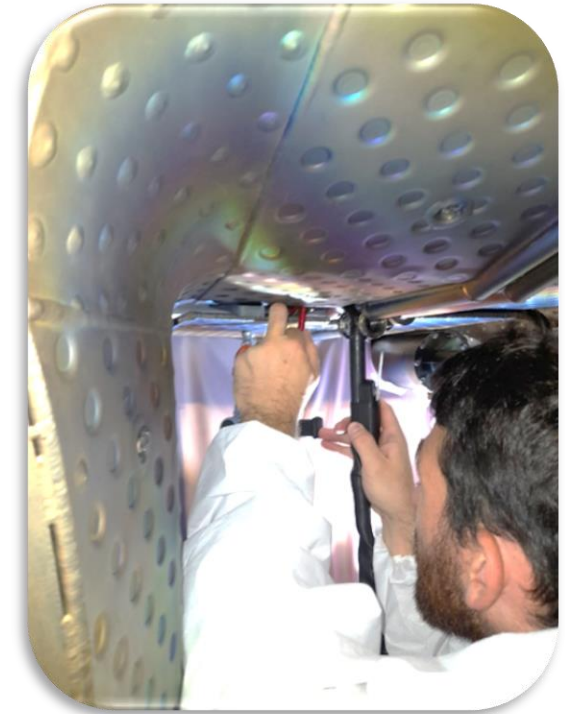
Induction brazing on Baffle connections
