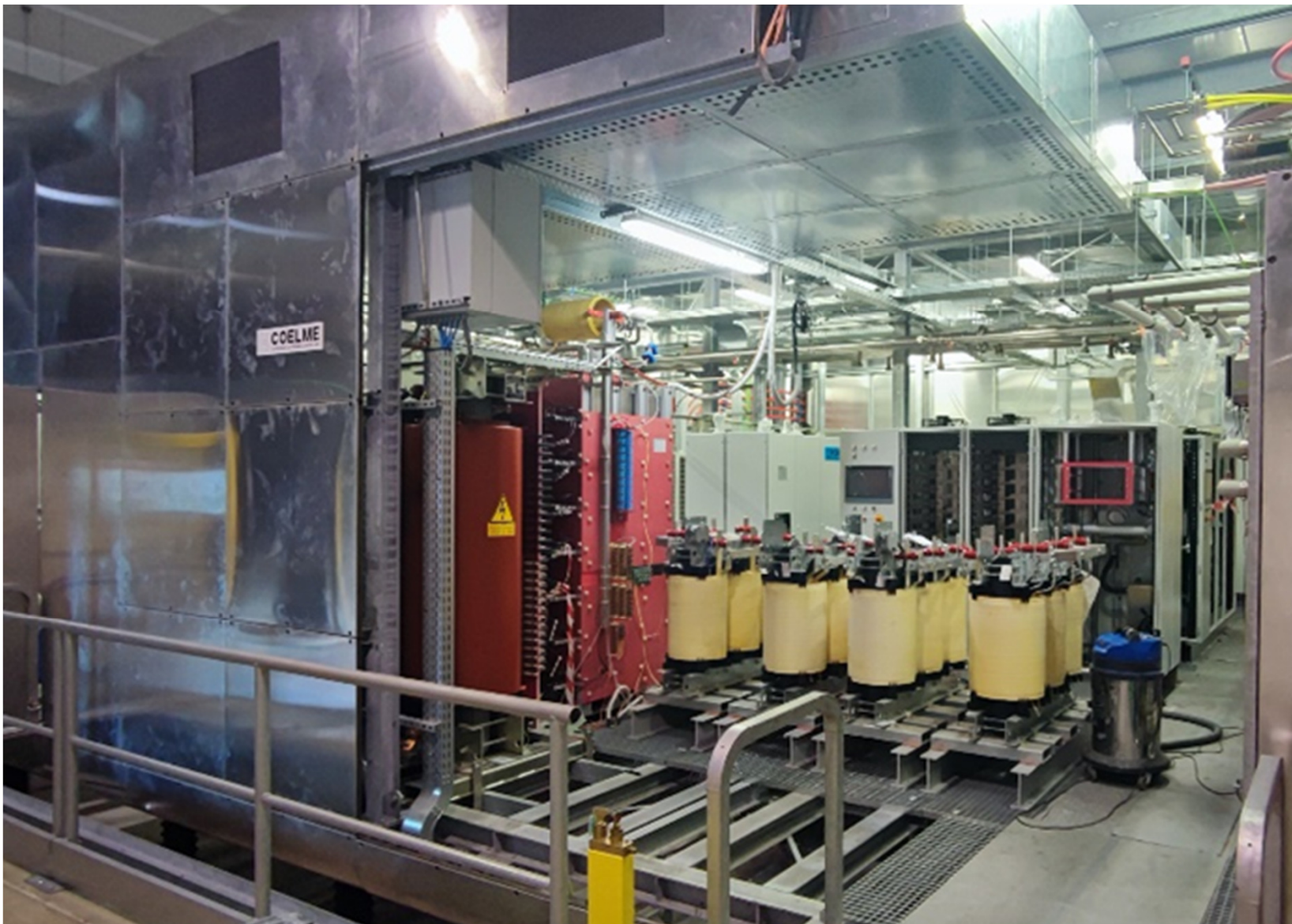
Completing SPIDER configuration: ongoing installation of new vessel module with NEG pumps and new RF solid-state amplifiers
