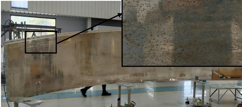
Galvanic corrosion in two panels
