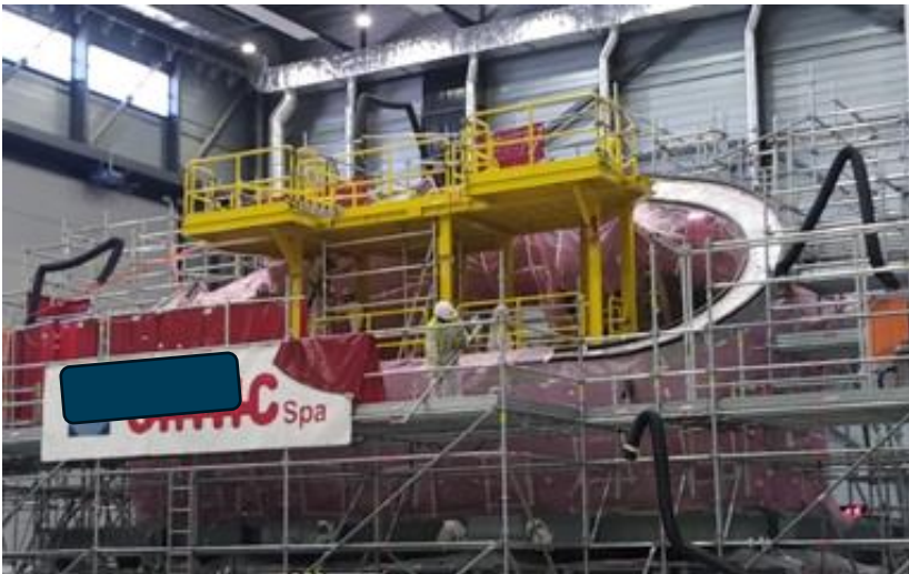
Sector repair in horizontal position
