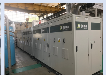
Left: TF magnet first winding pack. Right: TF power supply installed in the cold coil test facility in Frascati where all the Nb3Sn coils will be tested.
