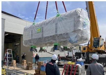
Unloading to the LIPAc Building
