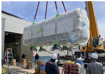
Unloading to the LIPAC Building
