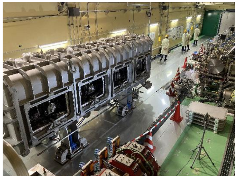
In the accelerator vault
