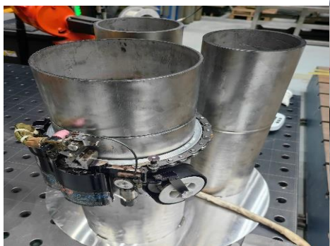
Automatic TIG welding of \varphi 300 \times 25 tubes in confined space
