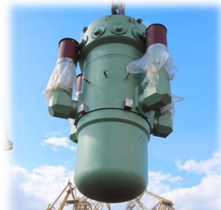
Installing the RITM-200 steam generating unit
