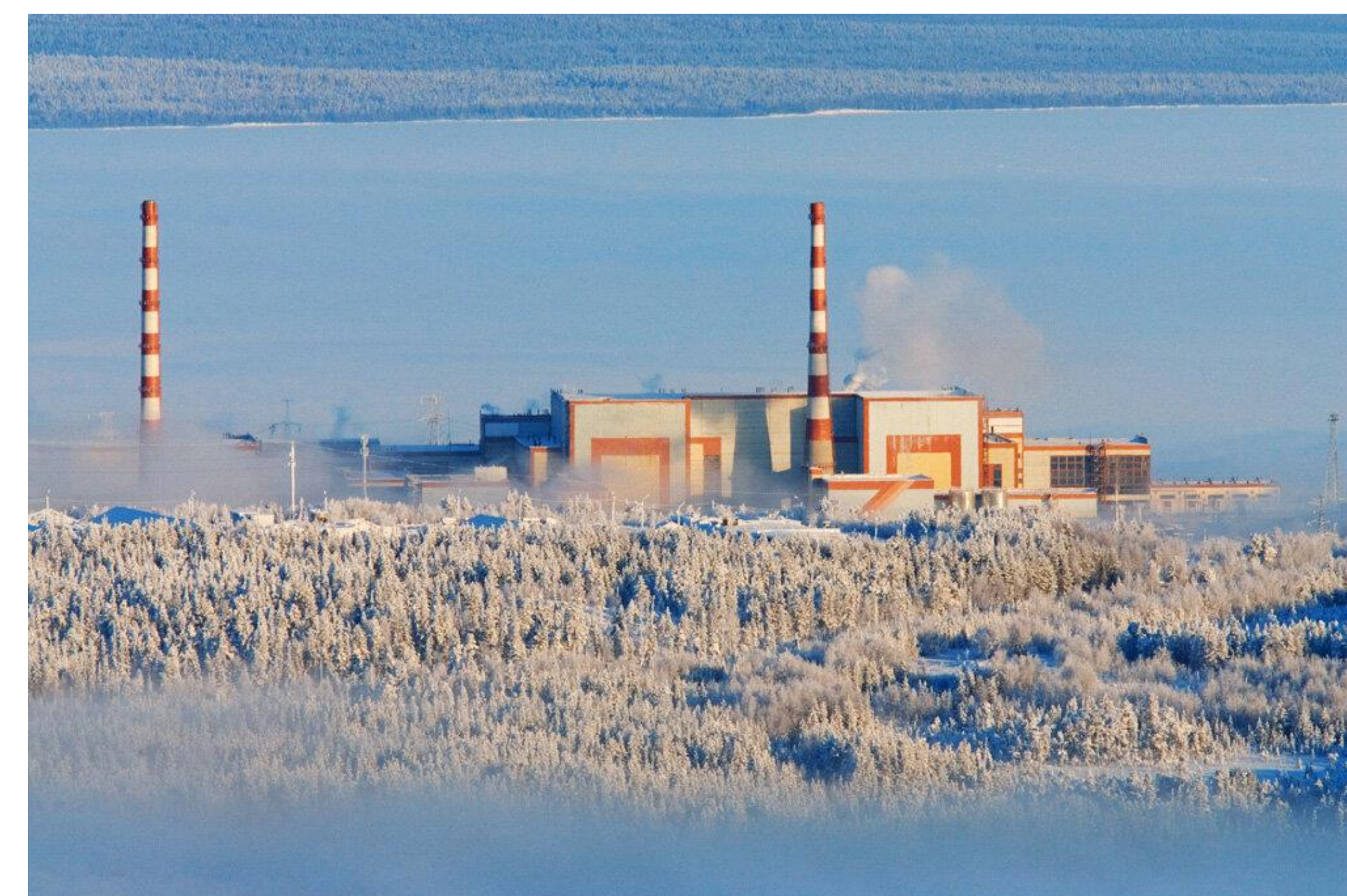
Kola NPP The northernmost nuclear power plant in Europe
