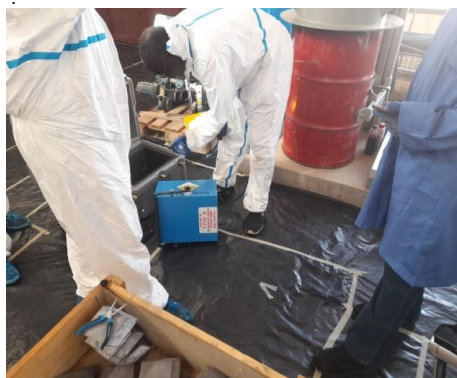
Dismantling of Source
