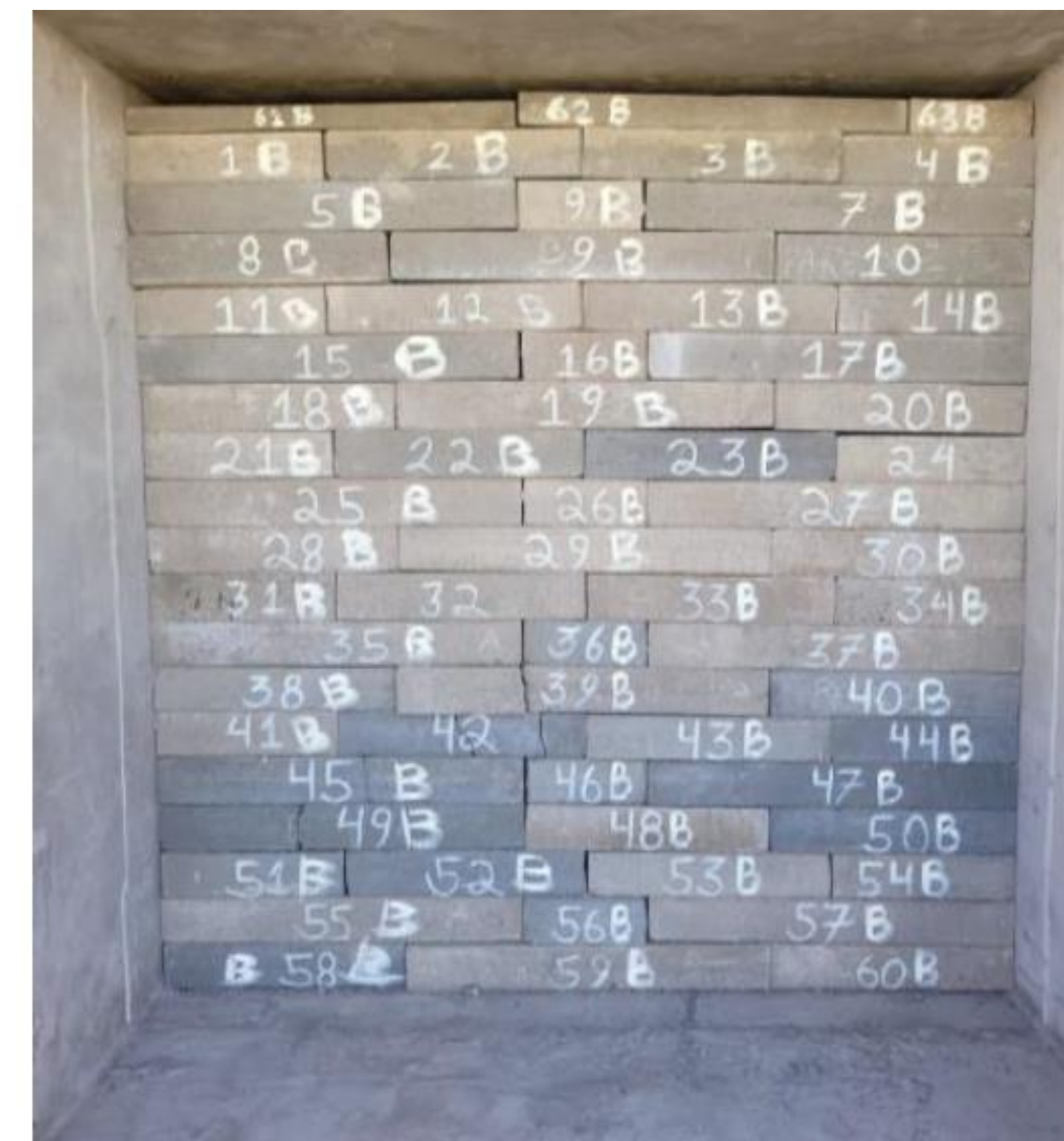
Figure 1: Characterization of bunker's concrete blocks during decommissioning process in Cyclotron facility in Brazil (CNEN collection)
