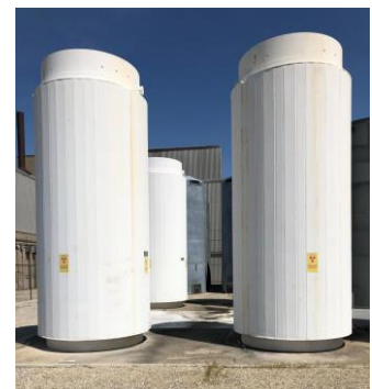
Left: CASTOR X/28 casks and Right: HI STAR 100 casks at Koeberg NPP.
