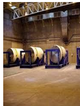
Left: CASTOR X/28 casks and Right: HI STAR 100 casks at Koeberg NPP.
