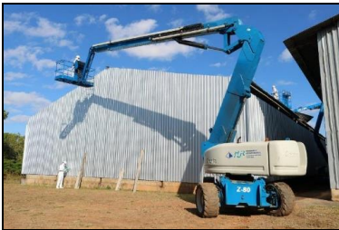
Figure 1. Infrastructure improvements in the Shed C-07.
