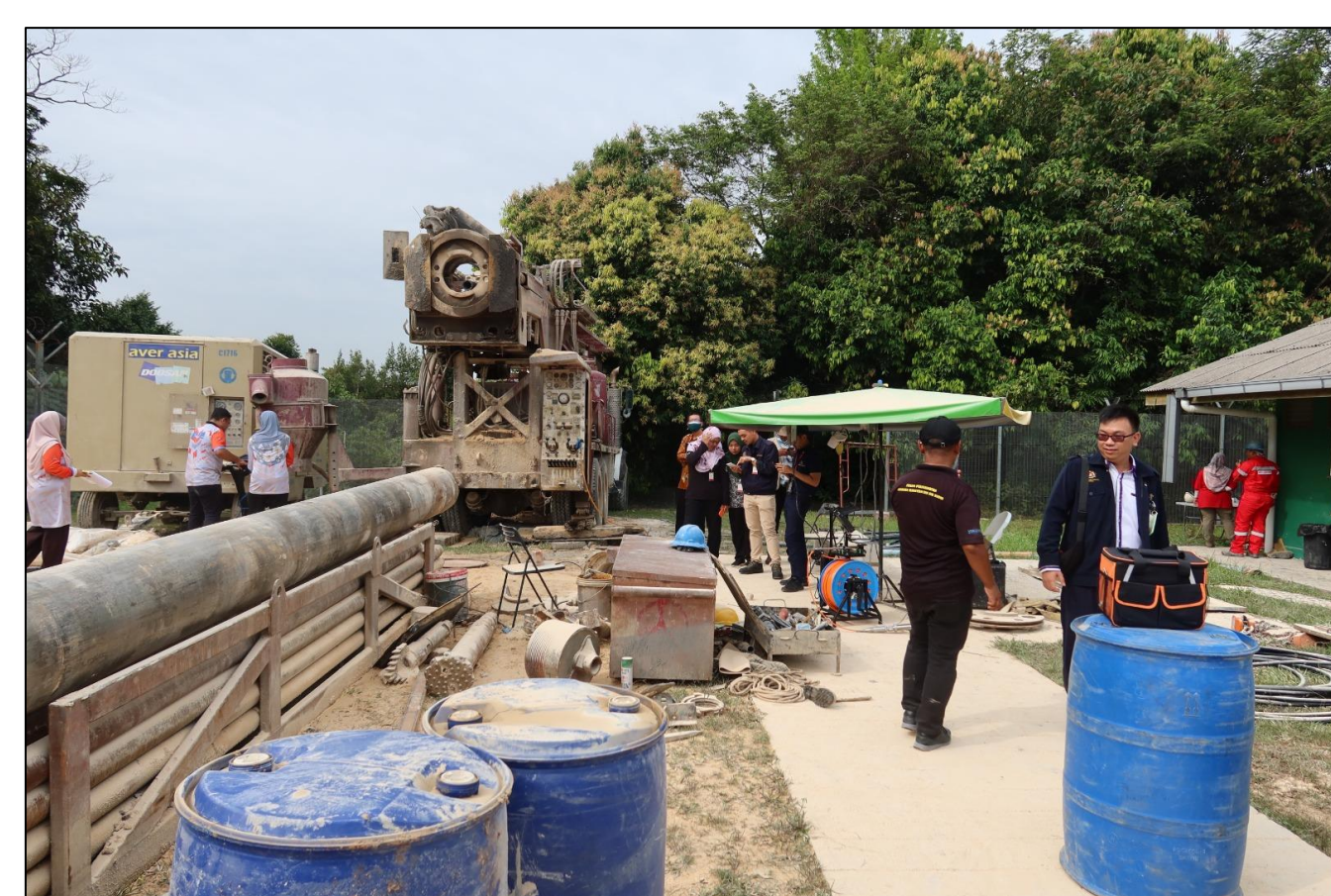
Fig. 3: Technical visits to the project site
