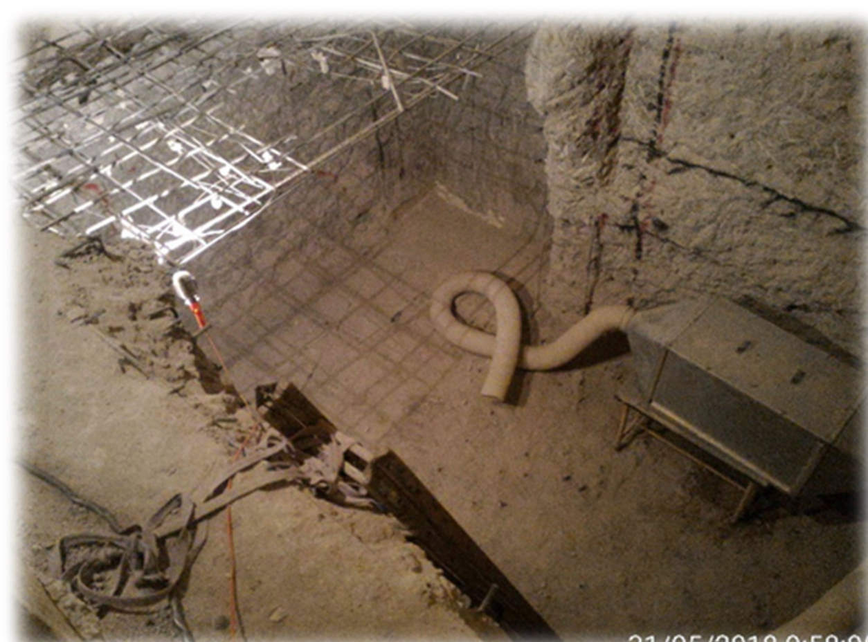
Reactor box after decontamination
