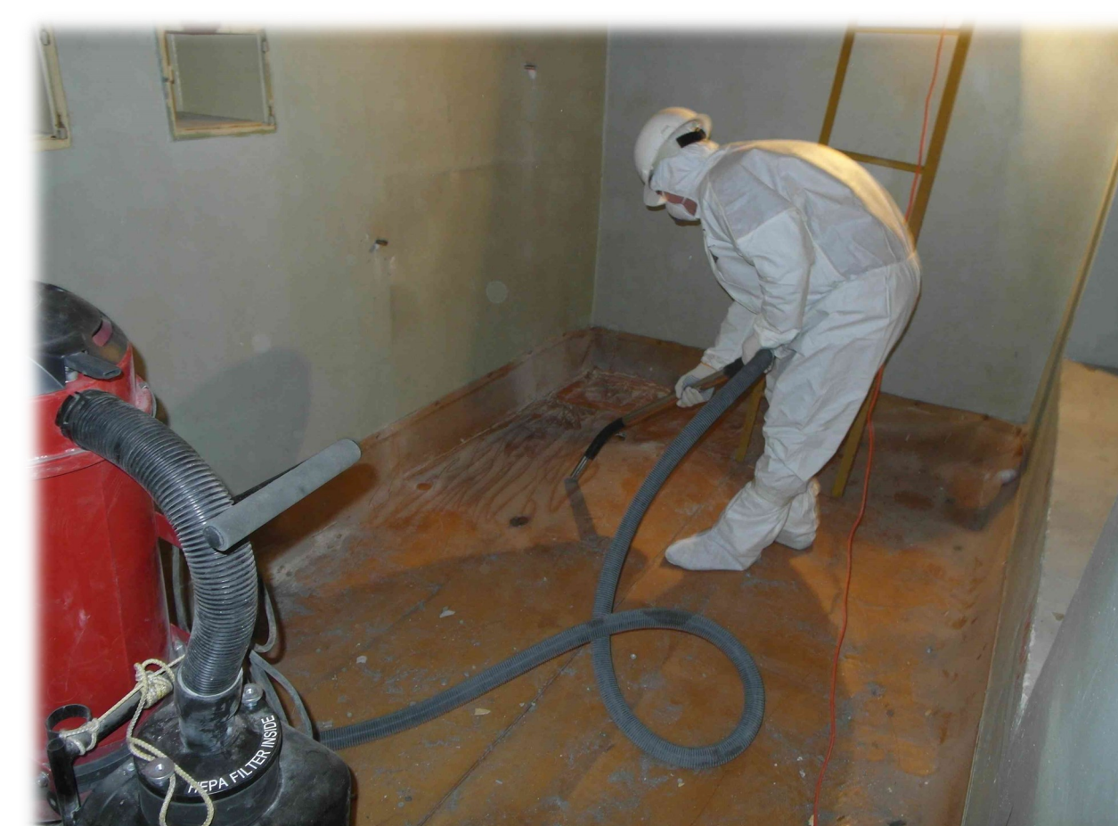
Decontaminating hot cell in a reactor building
