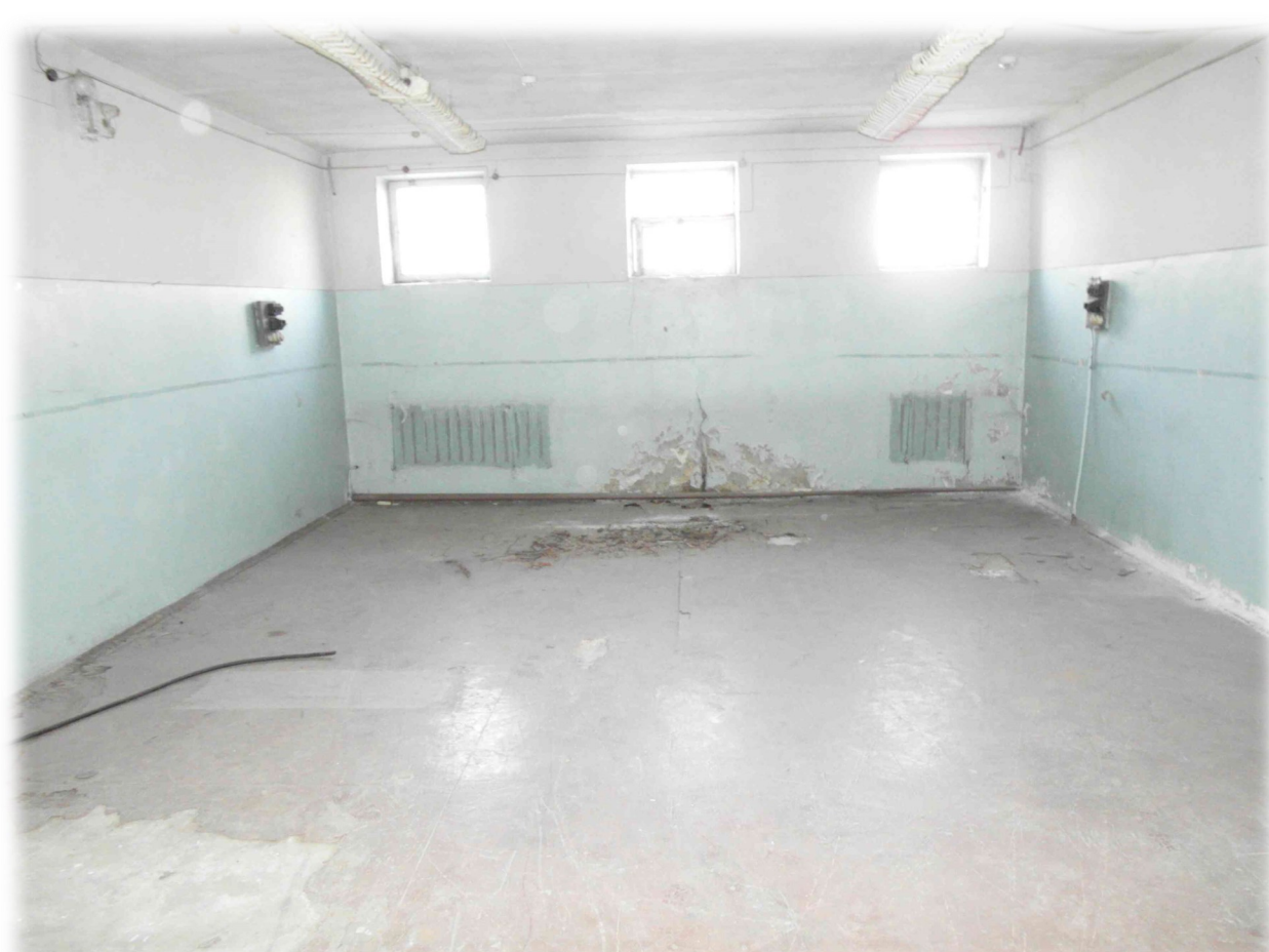
Decontaminated laboratory room in a reactor building
