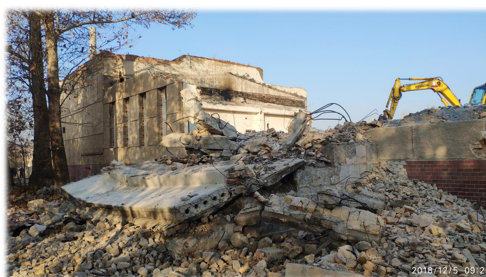
Reactor building demolishing
