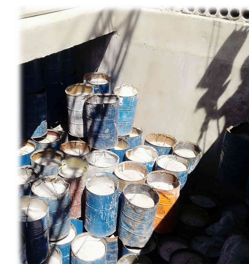
Radwastes from the RTC placed at the Republican Radioactive Waste Disposal Facility (RRWDF)
