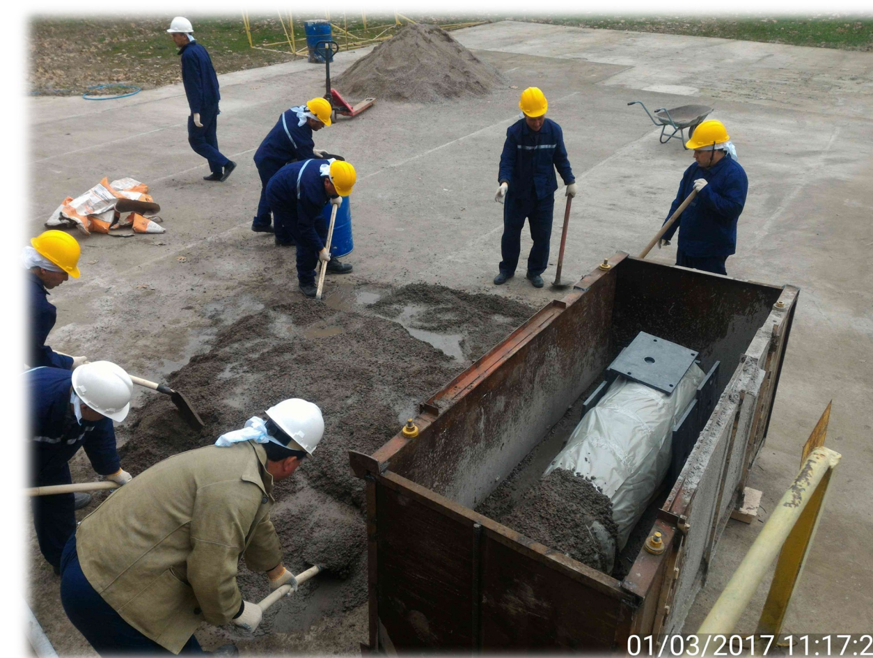
Covering reactor vessel with concrete
