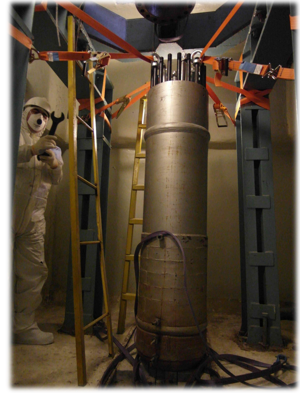
IIN-3M reactor vessel
