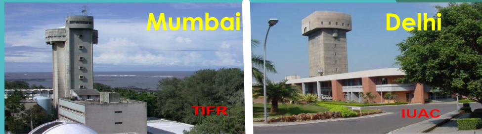
Two heavy ion accelerators installed in late 80's
